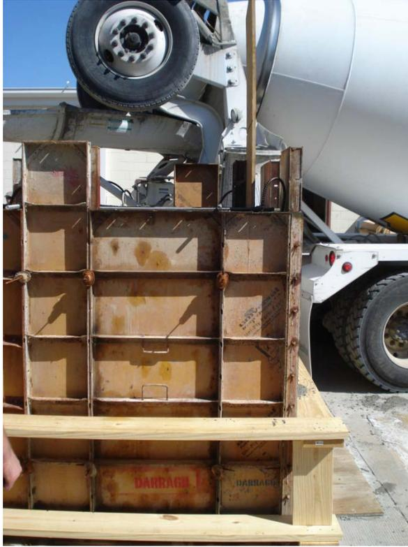
**Figure 6.21: Ready-Mix Truck Casting Box Culvert # 2**
