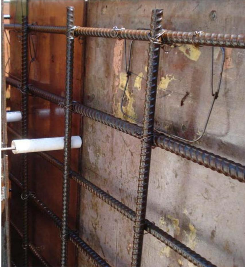
**Figure 6.6: Completed Inner Structure of the First Box Culvert**
