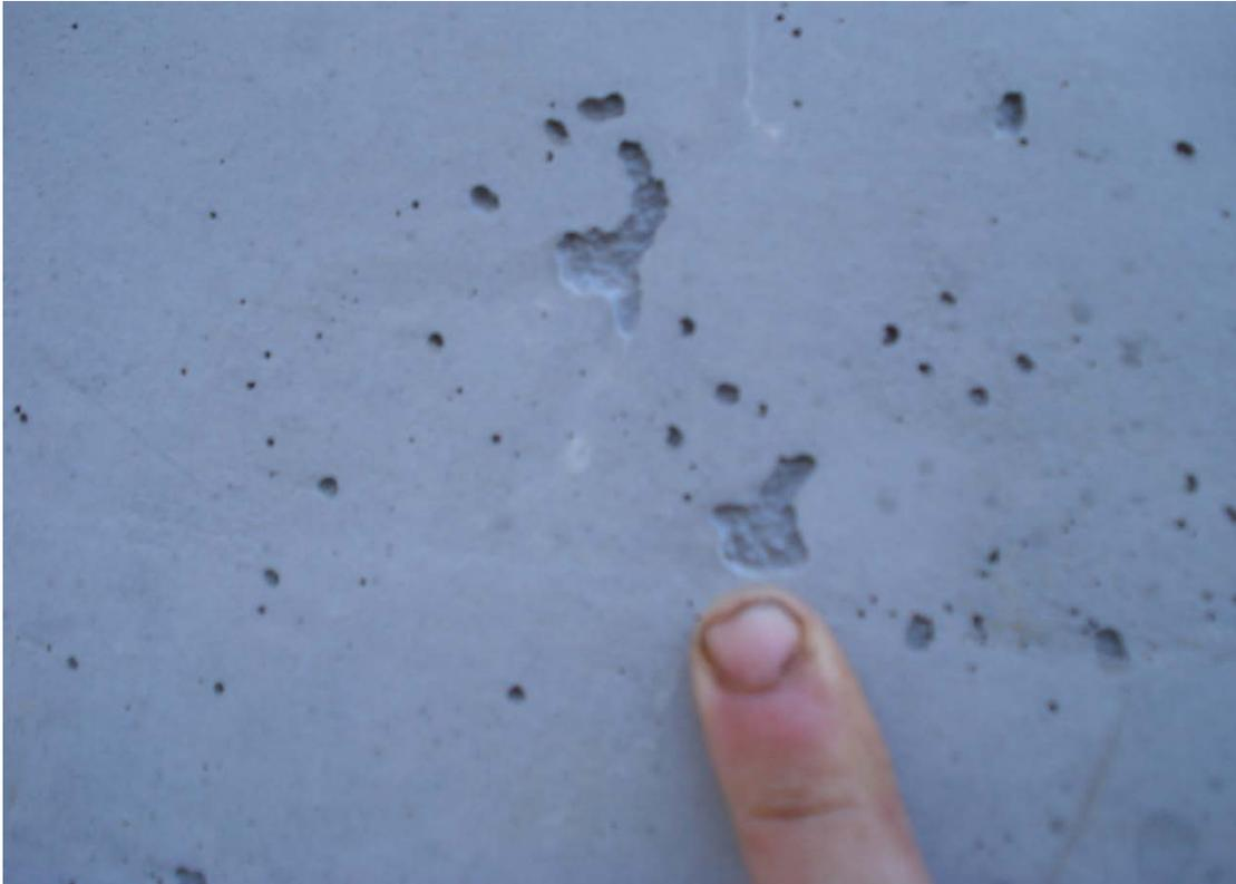
**Figure 6.18: Localized Surface Blemishes Present on Box Culvert # 1**
