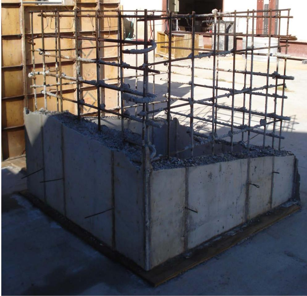
**Figure 6.16: Smooth Finish of Box Culvert # 1**
