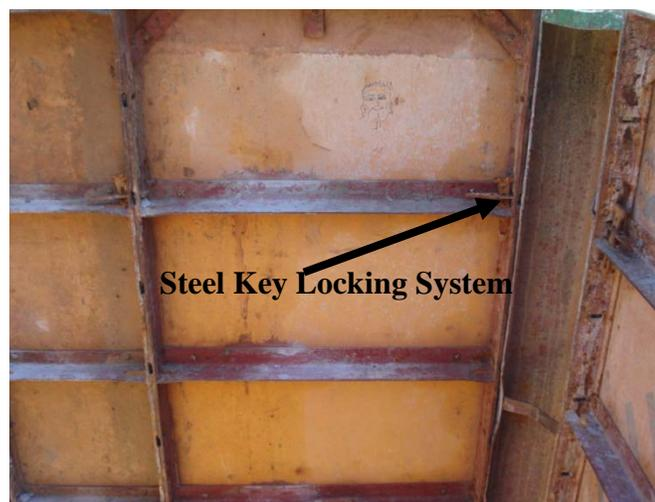
**Figure 6.3: Steel Key Locking System**
