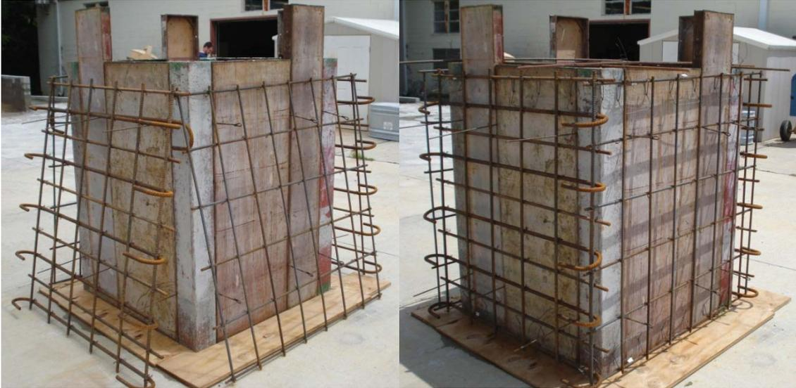
**Figure 6.5: Rebar Cages and the Corresponding Rebar Matrix**
