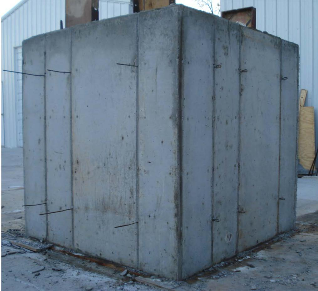
**Figure 6.24: Completed Box Culvert # 2 after Removal of Formwork**
