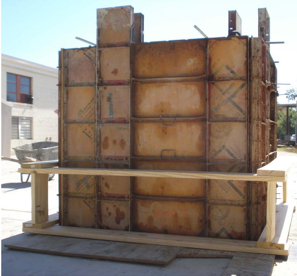
**Figure 6.20: External Lateral Reinforcement that was provided for Box Culvert # 2**
