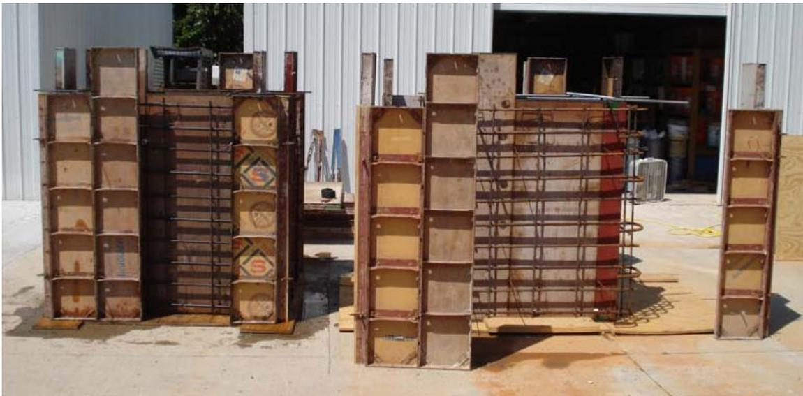
**Figure 6.7: Reinforced Box Culverts near Completion**
