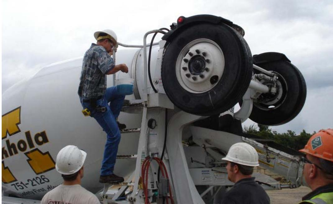
**Figure 6.10: Adding HRWR to Trial Batch # 1a**
