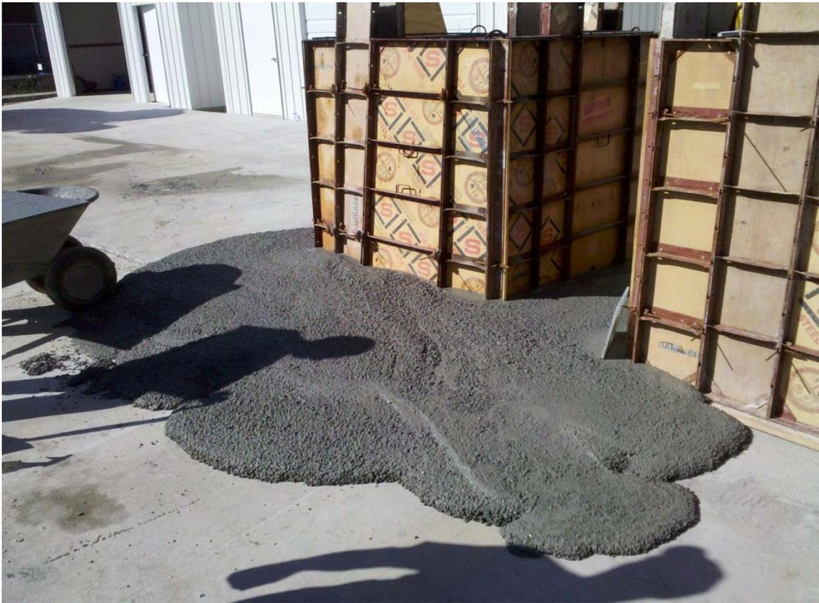
**Figure 6.14: Formwork Failure in Box Culvert # 1**
