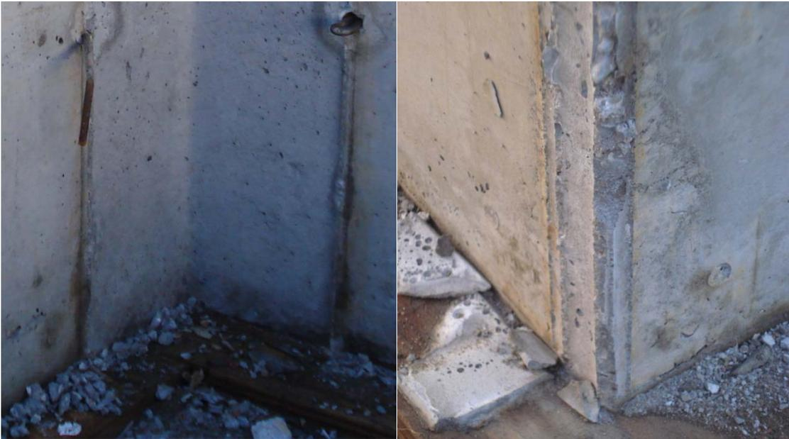
**Figure 6.17: Smooth Finish of Interior and Exterior Corners of Box Culvert # 1**
